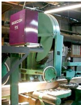
SEESAW installation at saw group 3
